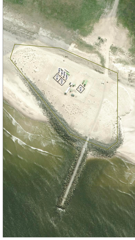
Figure 4: Location of the test cells and test pipes within the encapsulated area of Groyne 42.
